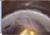
Picture of the tank's contaminated interior (The level of contamination inside the tank may vary depending on the number of years of the tank use.)
